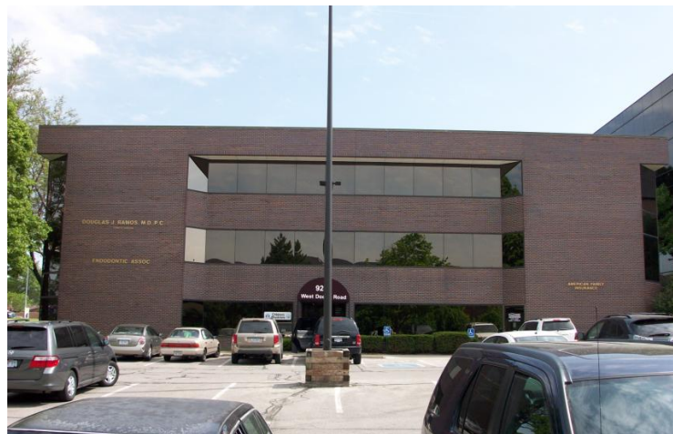
Figure 4-1: Building outside look
